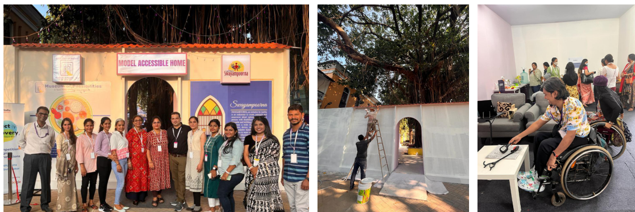
TARA, MoP and Anand Niketan team; Construction of the house; Attendees exploring the house (from left)
