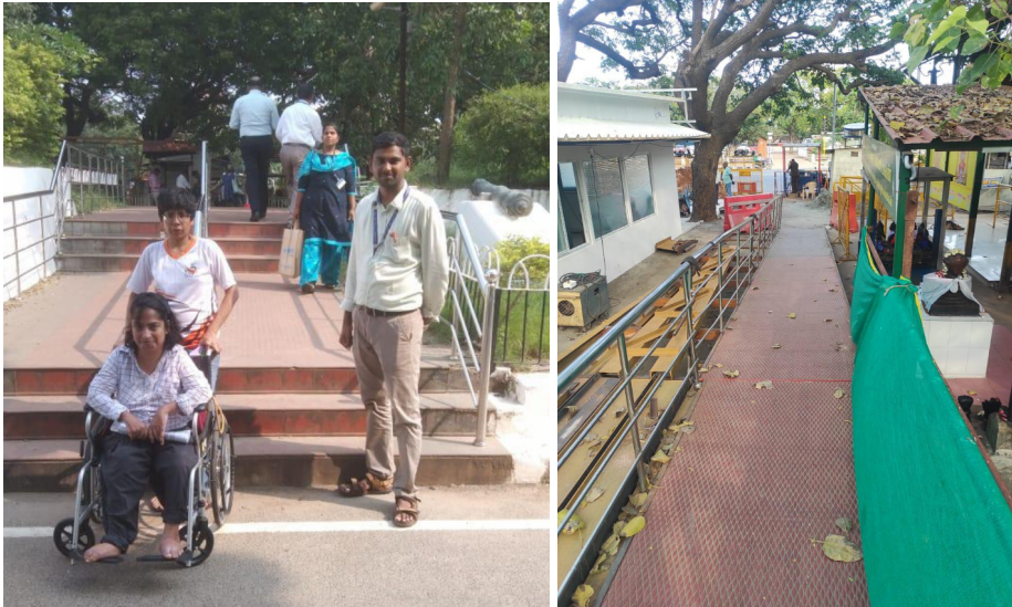
Before: The condition of the entrance at the Secretariat (To the left) After: The successful implementation of an accessible ramp (to the right)
